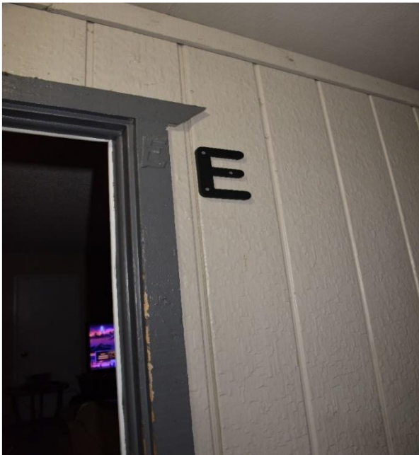
FIS Photo: Doorframe of Apartment E with door open.
